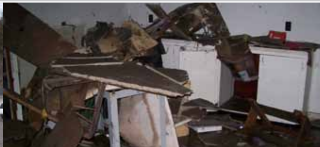
Damage to the inside of the funeral home.
