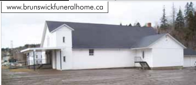
Brunswick Funeral Home, located in Perth-Andover, N.B., after the flood that hit them last March.
